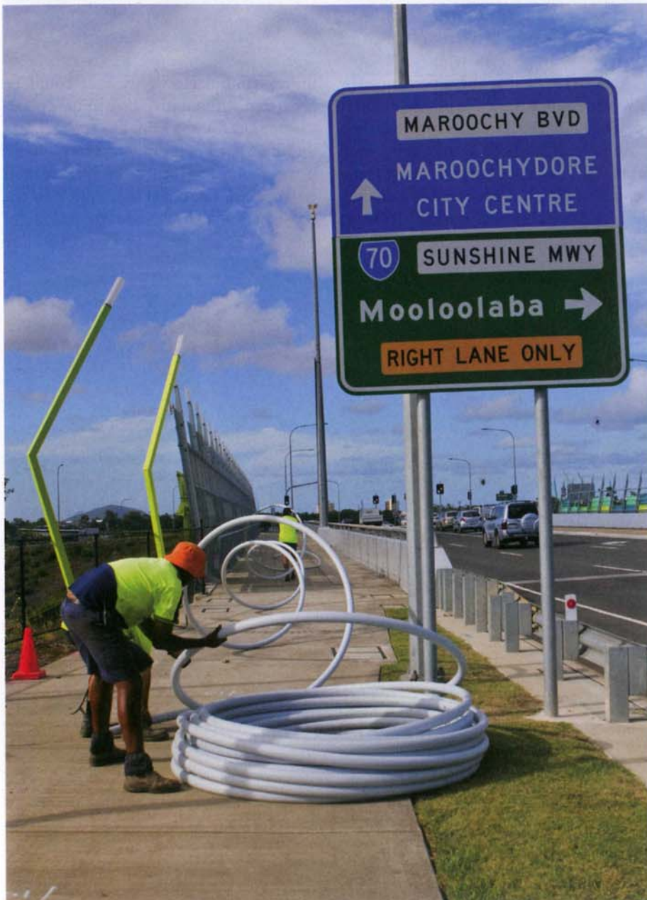
A worker installing an optical fibre conduit on Queensland's Sunshine Coast.
