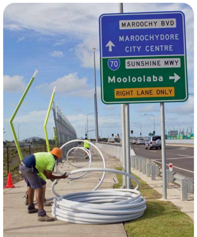
Optical fibre conduit being installed on the Sunshine Coast.
